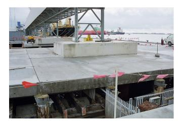
The slabs, each weighing over 20 tonnes and with a compressive strength of 40 MPa, were installed in an area exposed to saltwater, bulk chemicals, and fertilizers. Positioned in the splash zone, these slabs are subjected to constant wear and chemical exposure from off-loading operations at the wharf. The conditions demanded a concrete solution capable of providing long-term durability and protection against water ingress, chloride penetration, and chemical attacks.
